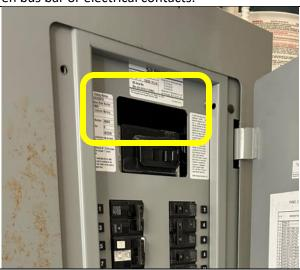
Please install a panel breaker filler plate to prevent inadvertent contact with a live bus bar or electrical contacts.
